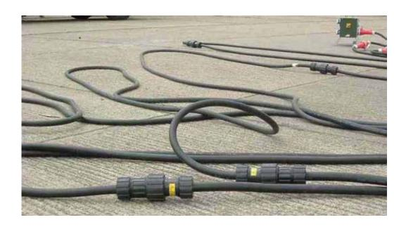
LUGIT is a safe and efficient to make temporary connection / extensions of single core power cables that are pre-terminated with copper lug terminals.
